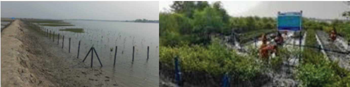
Figure 7. Success of fenced embankment reconstruction
