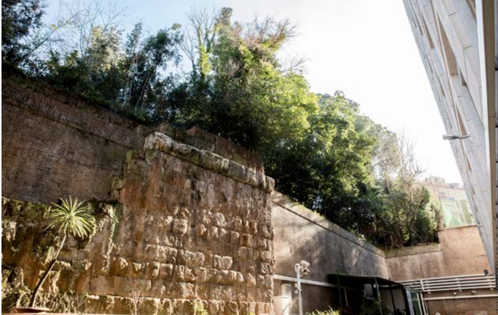
Roman terrace wall made of tuff and travertine in opus quadratum format from the second century BCE visible behind building C in the FAO complex.
